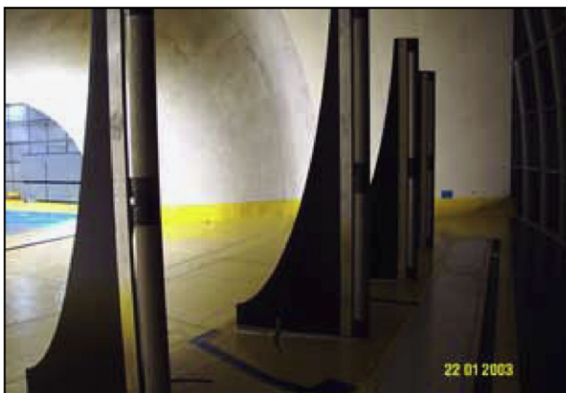
Fig. 9. (b) some views of the final TGS in operation since January 2003.
