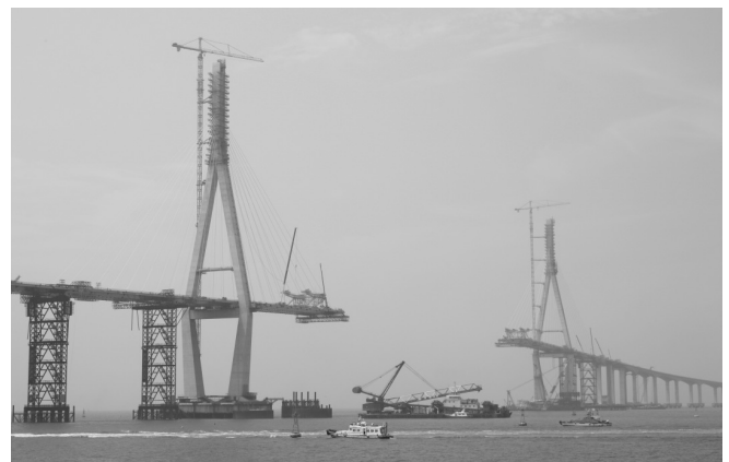
Fig. 2: construction of the Incheon bridge in South Korea.
